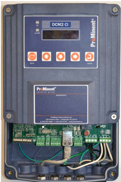
Interior of DCM 200 controller
