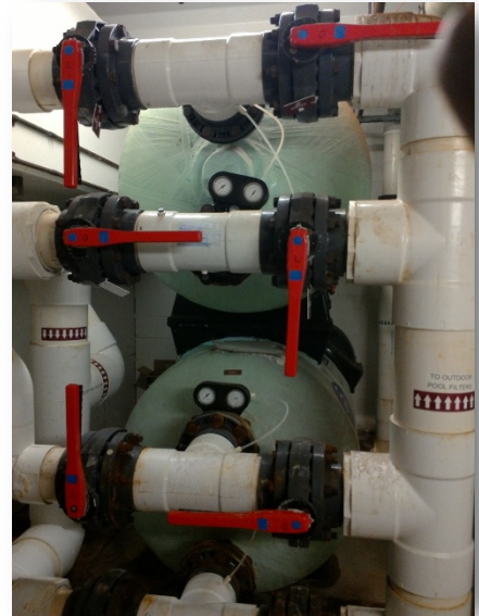
BEFORE: Two Wasteful Filters per Pool Plus Congested Space
