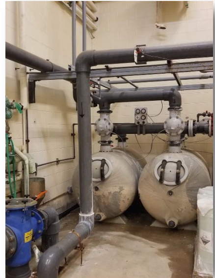
BEFORE: Two Wasteful Sand Bed Filters
